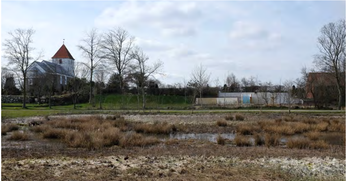
Fig. 1: Action D3 - Transformed abandoned house in Thisted Municipality, 2014.
